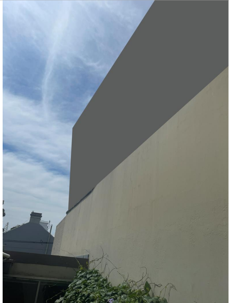
North facing master bathroom - obscured
