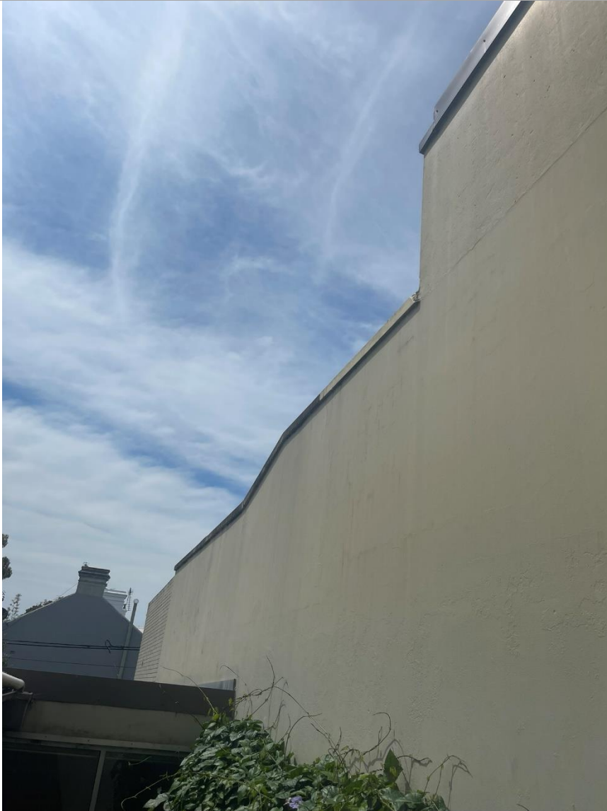
North facing master bathroom - existing
